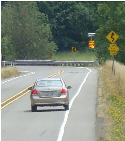
In-Radar Advanced Stats in use in two year CTRE study on dangerous road curves in the US
